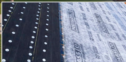
Complete Roof Replacement
