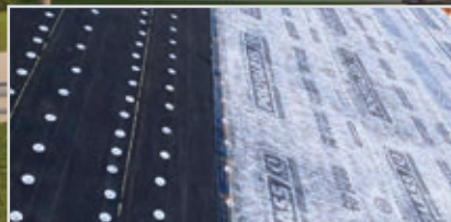
Complete Roof Replacement
