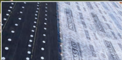
Complete Roof Replacement
