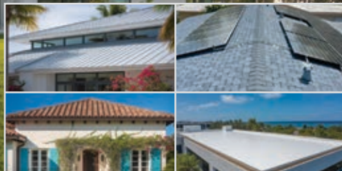
Metal, Shingle, Tile, and Flat Roof Systems
