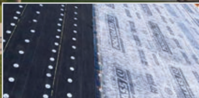
Complete Roof Replacement
