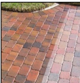
COMPLETE PAVER RESTORATION
