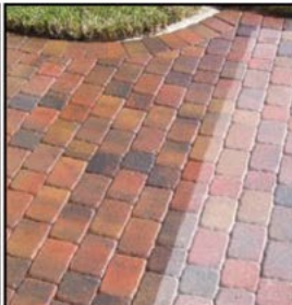
COMPLETE PAVER RESTORATION
