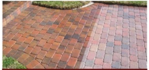
PAVER RESTORATION · ACID WASH · CHLORINE RINSE
