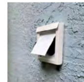
DRYER WALL VENT INSTALLS
