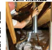
DRYER DUCT INSTALLS
