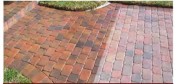
PAVER RESTORATION. COLOR BACK. TINTED SEALER
