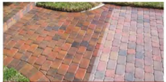
PAVER RESTORATION. COLOR BACK. TINTED SEALER
