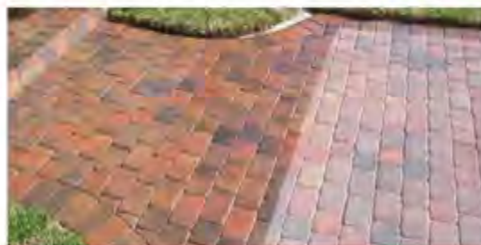
PAVER RESTORATION - ACID WASH - CHLORINE RINSE
